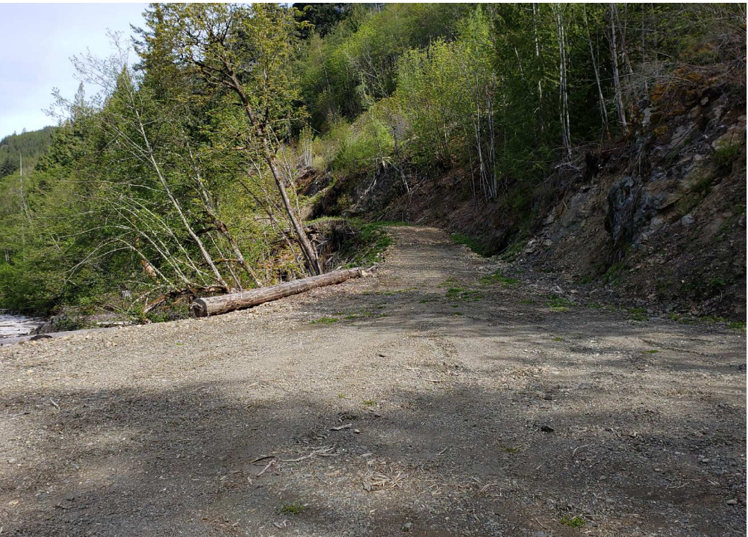
PHOTO #4 - VIEW FROM WORK AREA TOWARDS CAMP APPROACH
