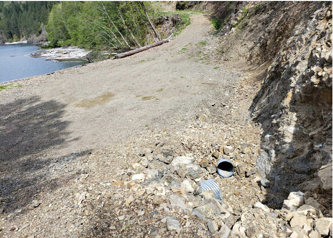
PHOTO #2 -VIEW OF EXISTING OIL SEPARATION CULVERTS
